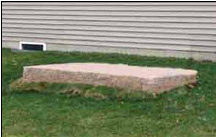
Figure 3-4. Concrete Pad Site
