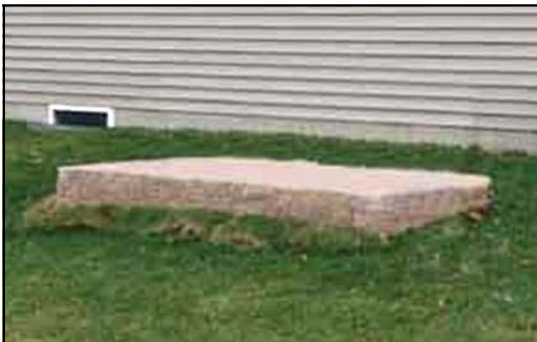
Figure 3-4. Concrete Pad Site
