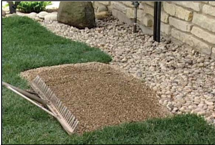
Figure 3-3. Compacted Gravel Site
